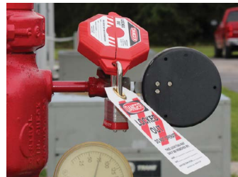
Gate Valve Handle Lockouts KDD471 For 2-1/2" - 5" handle
